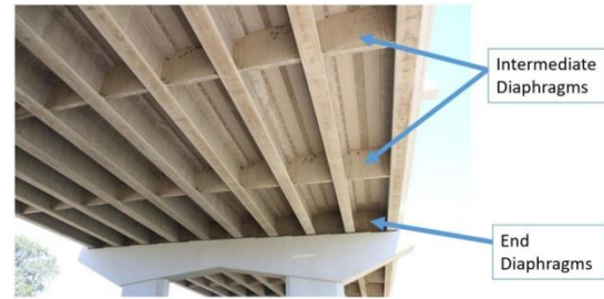
Fig. 3. : Intermediate and end diaphragms in a concrete bridge (Weeks 2011).
